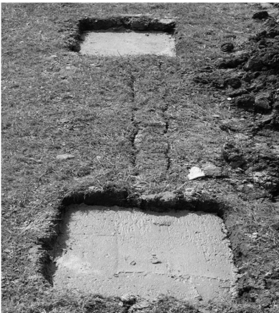
Typical Concrete Pad finish
